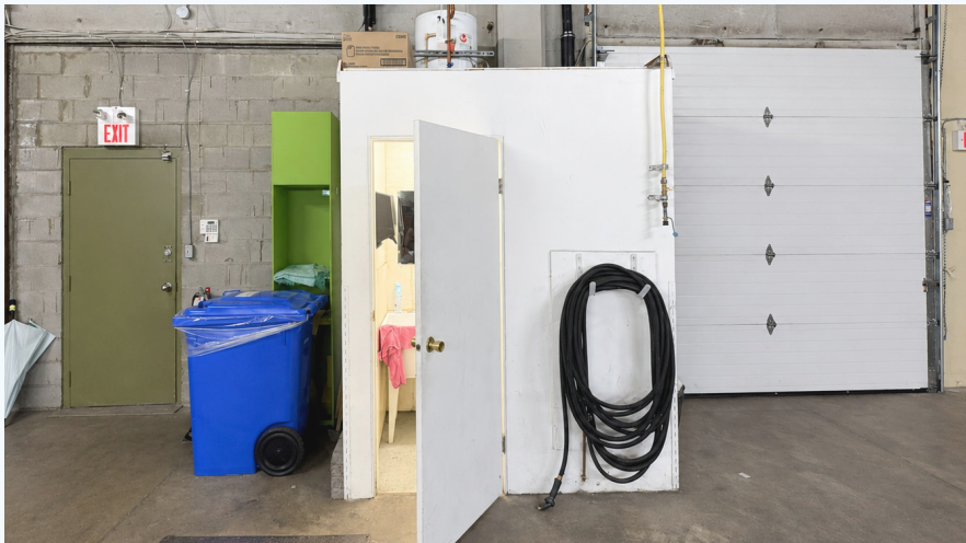
Rear Loading Bay
